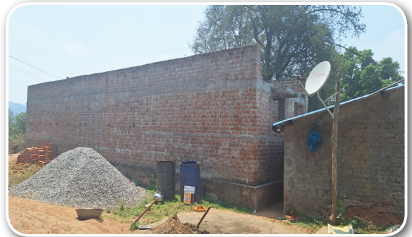
PMI Housing Project – Santhosh, Berhampur, Odisha.
